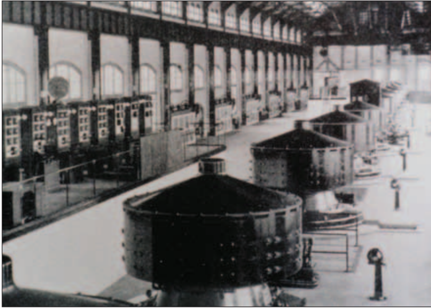
The AC electrical power system at Niagara Falls
